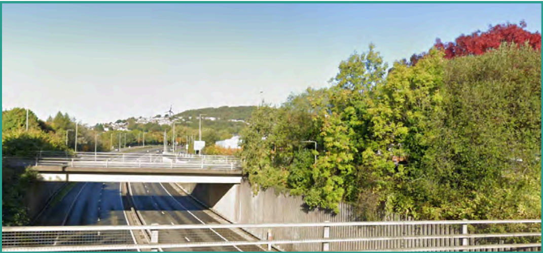
A470 Sainsbury's Roundabout
