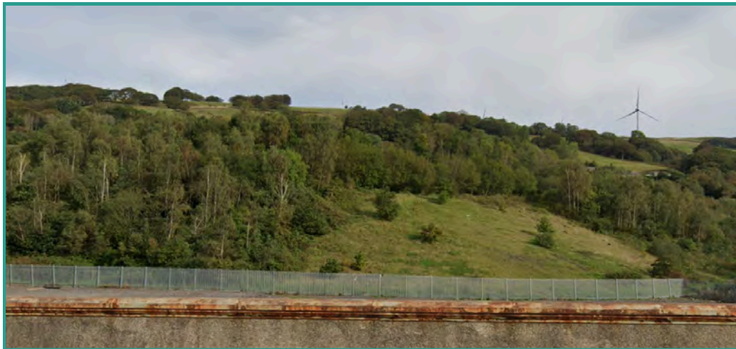
Llwyncelyn Road bridge (near the industrial estate)
